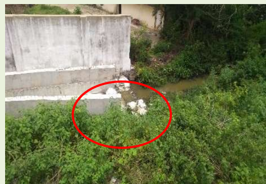
Figure-3.4 : Shortened weir at Mukkidi Cheruvu (23 August 2018)
